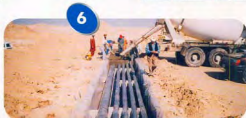
PVC Pipes Installed on an Infrastructure Project
