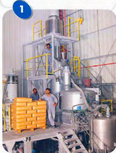
High Speed Mixing Plant
